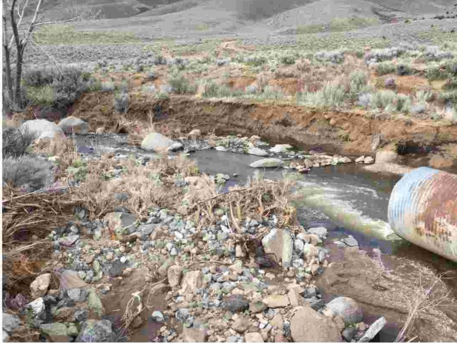
**Downstream damage to creek from Washed out Culvert**
